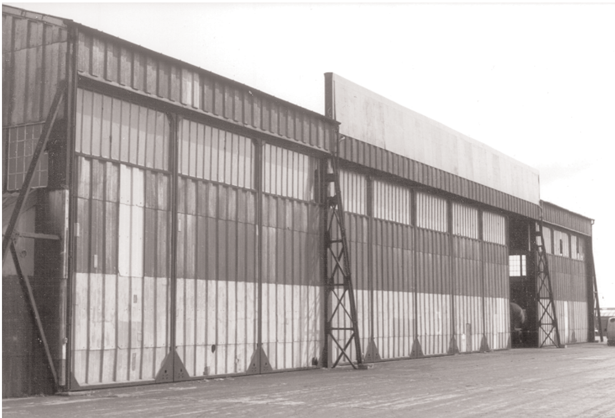
Type 'F' Admiralty Seaplane Shed at Jurby Airfield. One of many buildings identified as being of historic interest in a recent survey undertaken by the Manx Heritage Foundation
