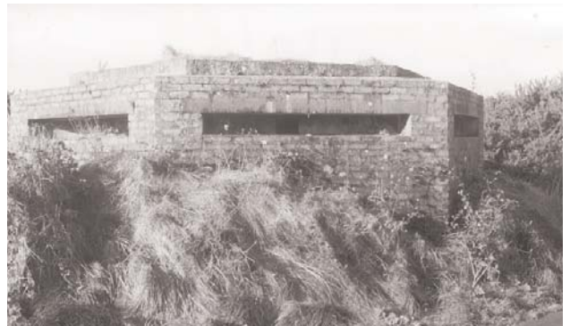
A 'Type 22' pill box - one of a number still surviving on the perimeter of Jurby Airfield giving an indication of the defence strategy of this important training site.
