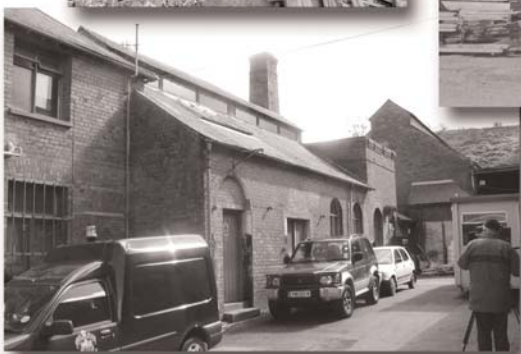
Lake Road - due for demolition
